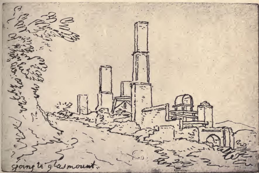
WORKS FOR COPPER MANUFACTURE WITH ACCOMPANY POWER. IN LLANGAVELACH PARISH NEAR SWANSEA.
