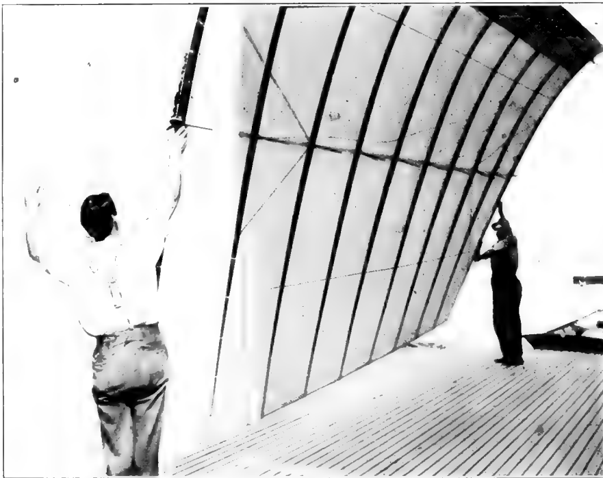
HOISTING WING OF FULL-SIZE AERODROME
