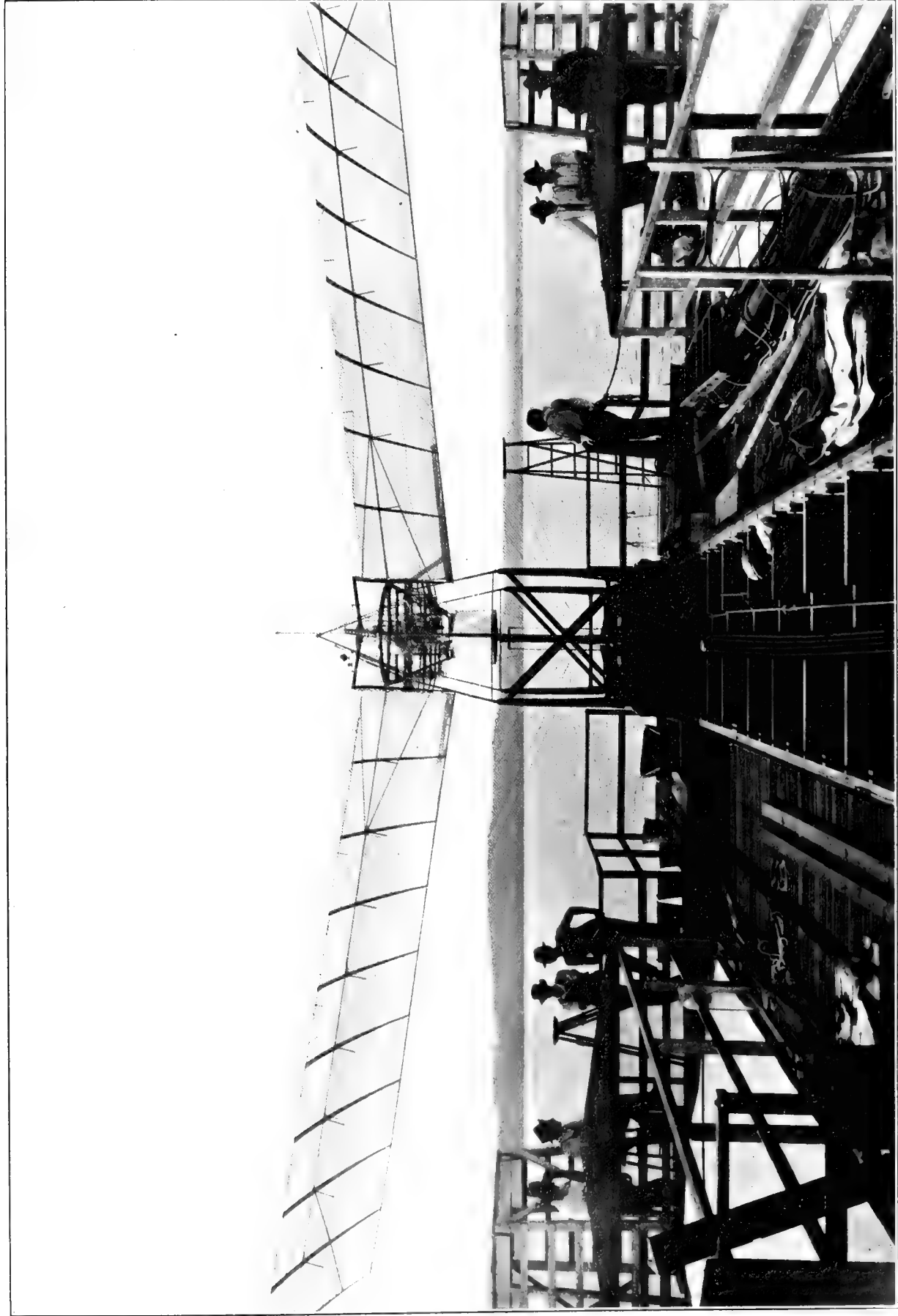
AERODROME ON LAUNCHING-CAR; FRONT WINGS IN PLACE. GUY-WIRES ADJUSTED
