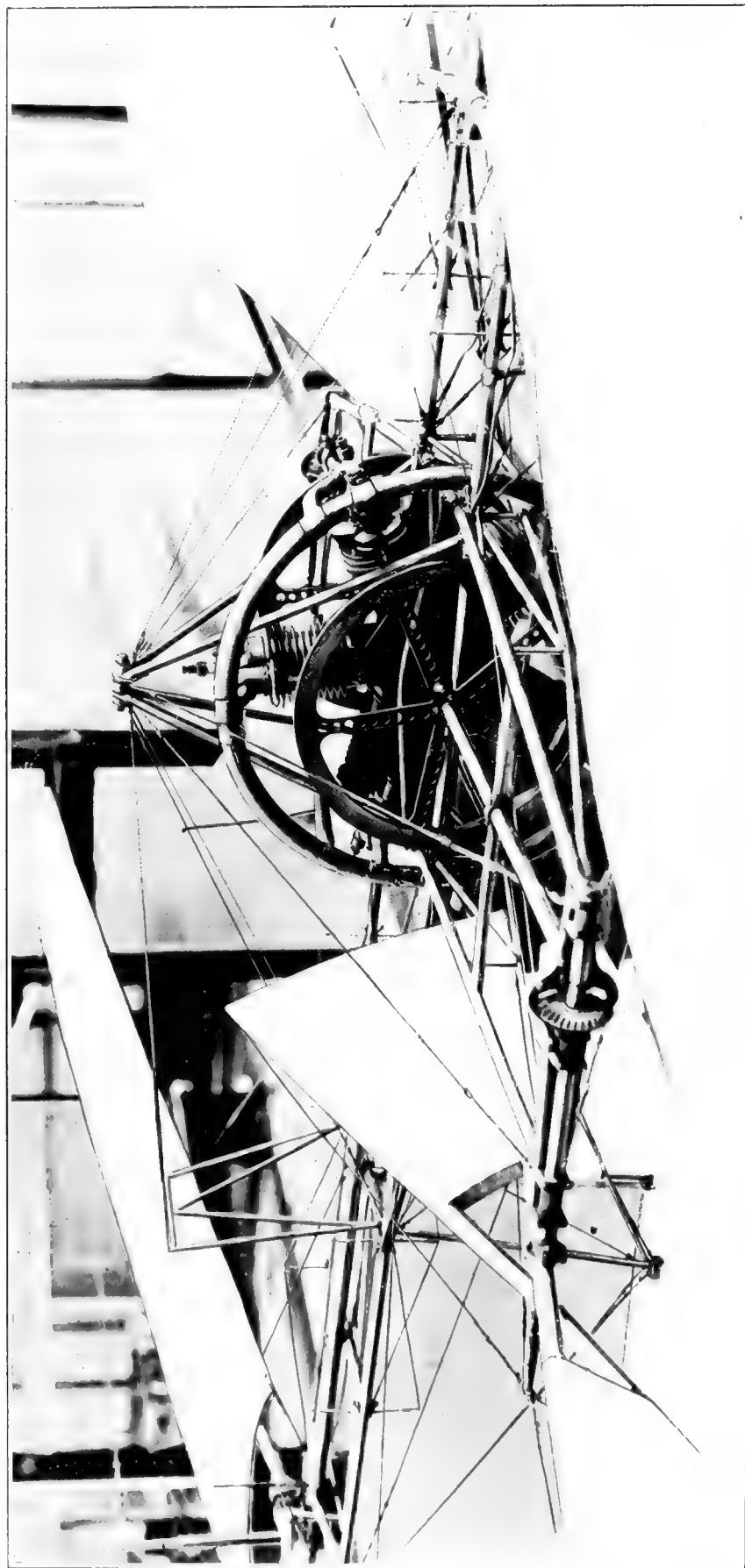
CYLINDERS OF ENGINE OF QUARTER-SIZE MODEL AERODROME
