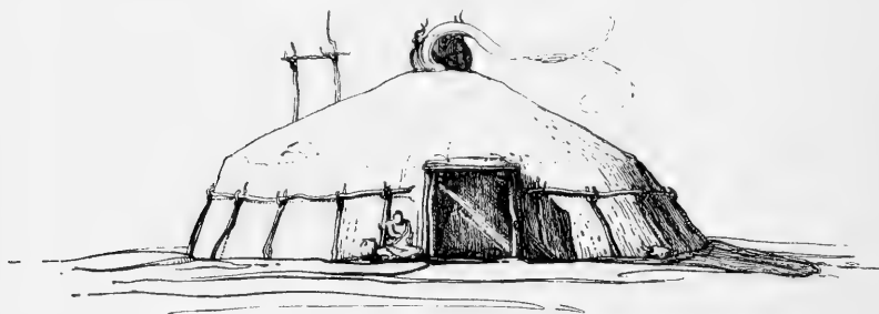
FIG. 27.—Exterior view of same historic Arikara earth lodge (reconstruction), Leavenworth site.
