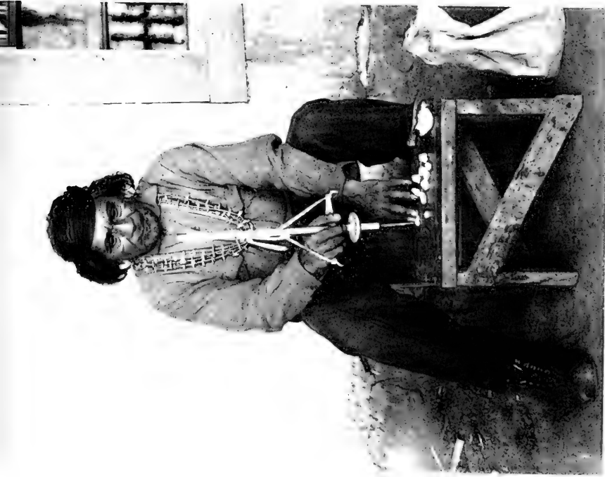
Zuni man drilling turquoise with pump drill. (Photograph by O. C. Havens, 1924.)
