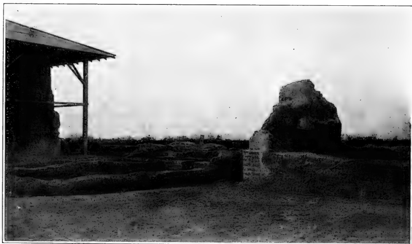
b View from same point after excavation
