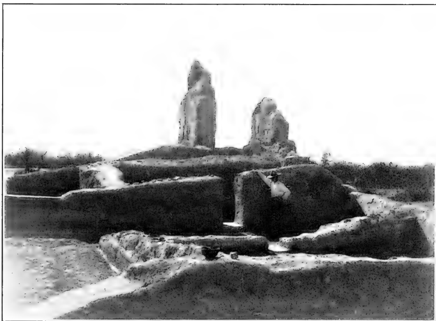
b View from north SOUTHWEST BUILDING
