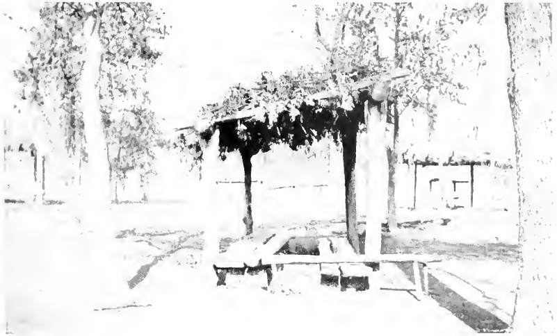
FIG. 48.—West cabin, Chiaha busk ground. Photograph by Swanton.
