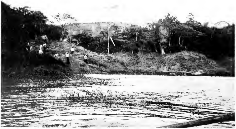
FIG. 70.—Rio Grande Reservoir, Canal Zone, showing workmen clearing the shores to prevent decaying vegetation from falling into the water. This is an old reservoir dating from the time of the French occupation. Photograph by Marsh.
