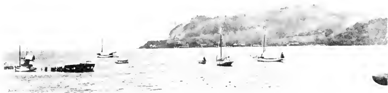
FIG. 75.—Porto Bello Bay, showing excavation in the mountain, where the rock used for the Gatun Dam was secured. Photograph by Busck.
