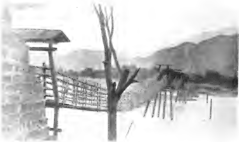
2. A great bridge made of large bamboo ropes or cables at Kuanshien, Szechuan, China.
