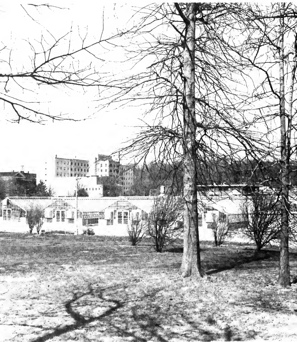
Five greenhouses leased from the United States Soldiers' and Airmen's Home by the Horticultural Services Division, Office of Plant Services, Support Activities.
