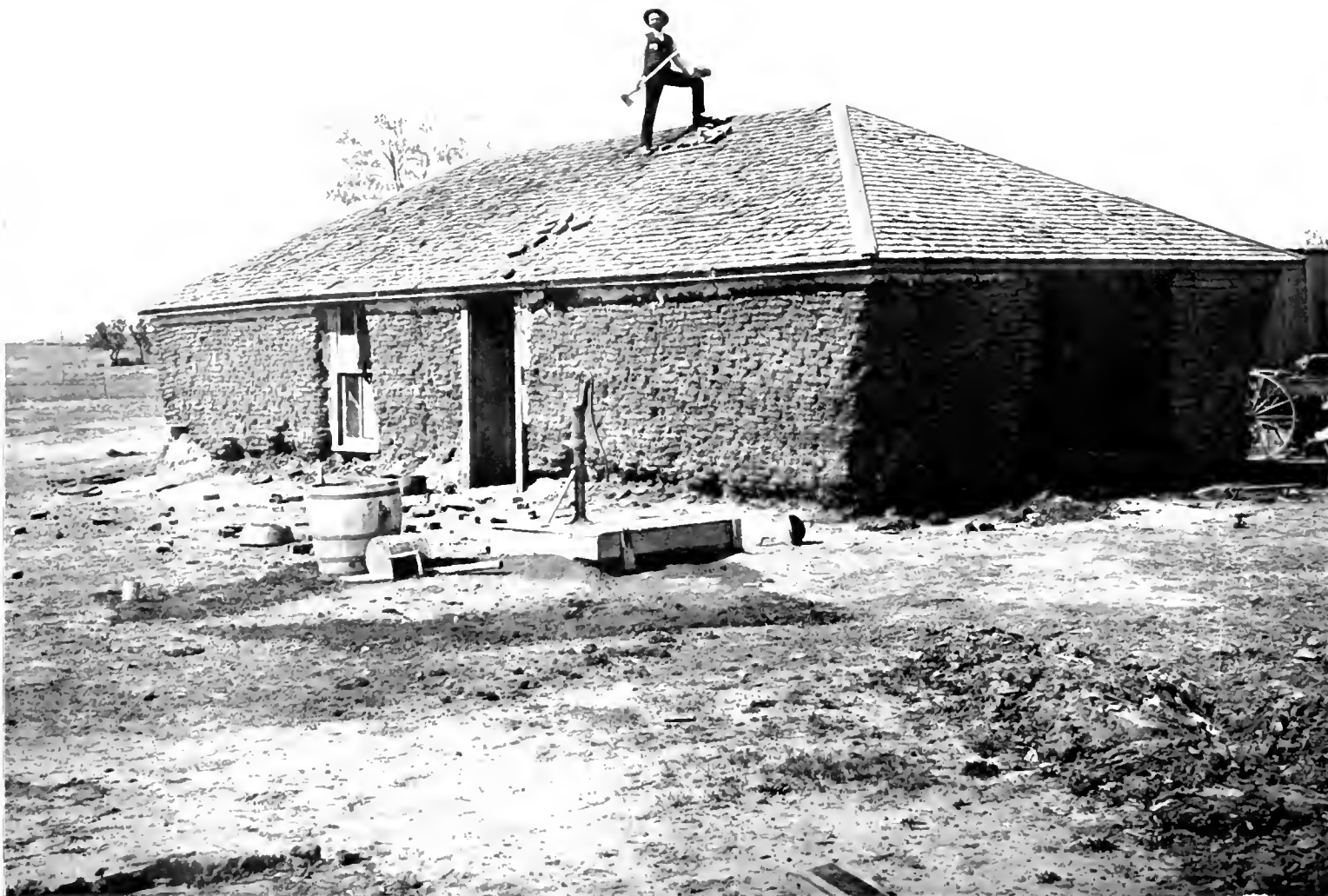
Shows the old Rymer sod house, built in 1886, Township 16, Range 20. It has served its purpose and is passing away. See opposite page now on same quarter section within 300 feet of old sods.
