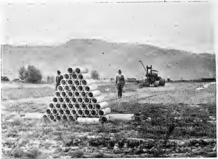
FIG. 20. — FIELD READY FOR LAYING TILE.
