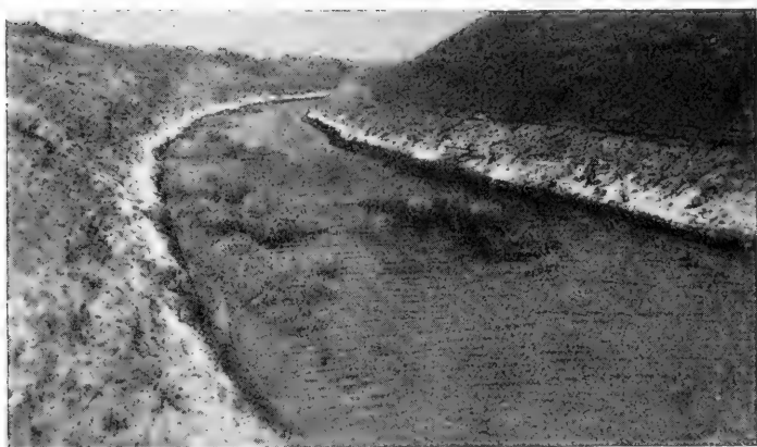
FIG. 22. — OPEN DITCH USED TO CARRY AWAY THE DRAINAGE WATER FROM A LARGE AREA. COVERED DRAINS EMPTY INTO THIS DITCH.
