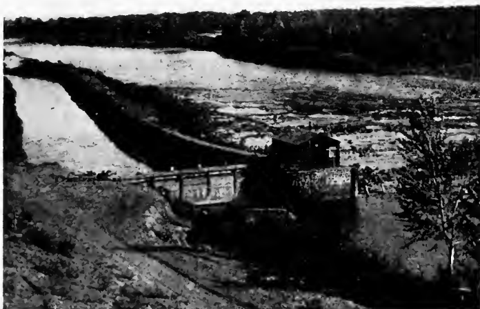
81. THE INTAKE OF THE SUNNYSIDE CANAL, YAKIMA VALLEY, WASHINGTON
