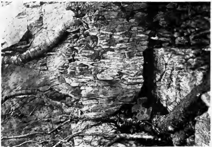
4. LEDGE BEING TORN APART BY THE GROWTH OF TREE ROOTS IN THE CREVICES
