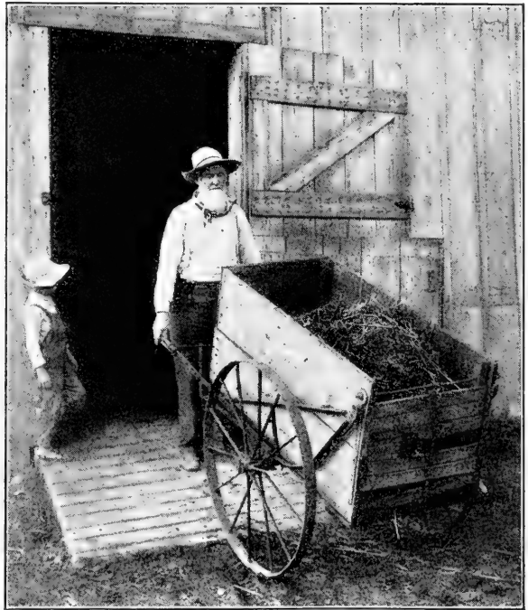
HOME-MADE DUMP CART TO MAKE STABLE WORK EASIER. 1
