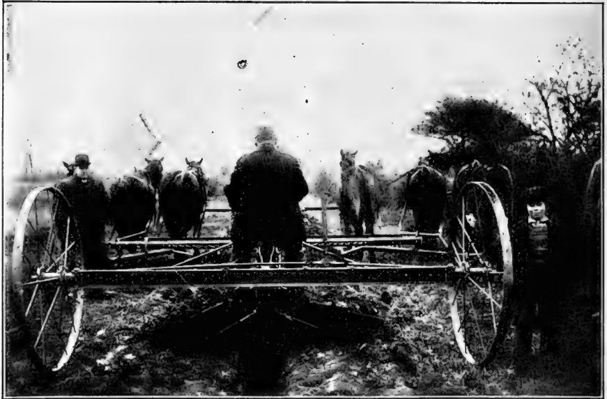
THE DITCHER IN OPERATION.
