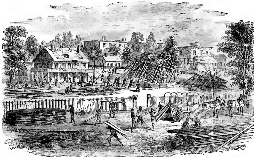
UNITED STATES SOLDIERS, AT ATLANTA, GA., TEARING DOWN BUILDINGS SHATTERED DURING THE BOMBARDMENT.
