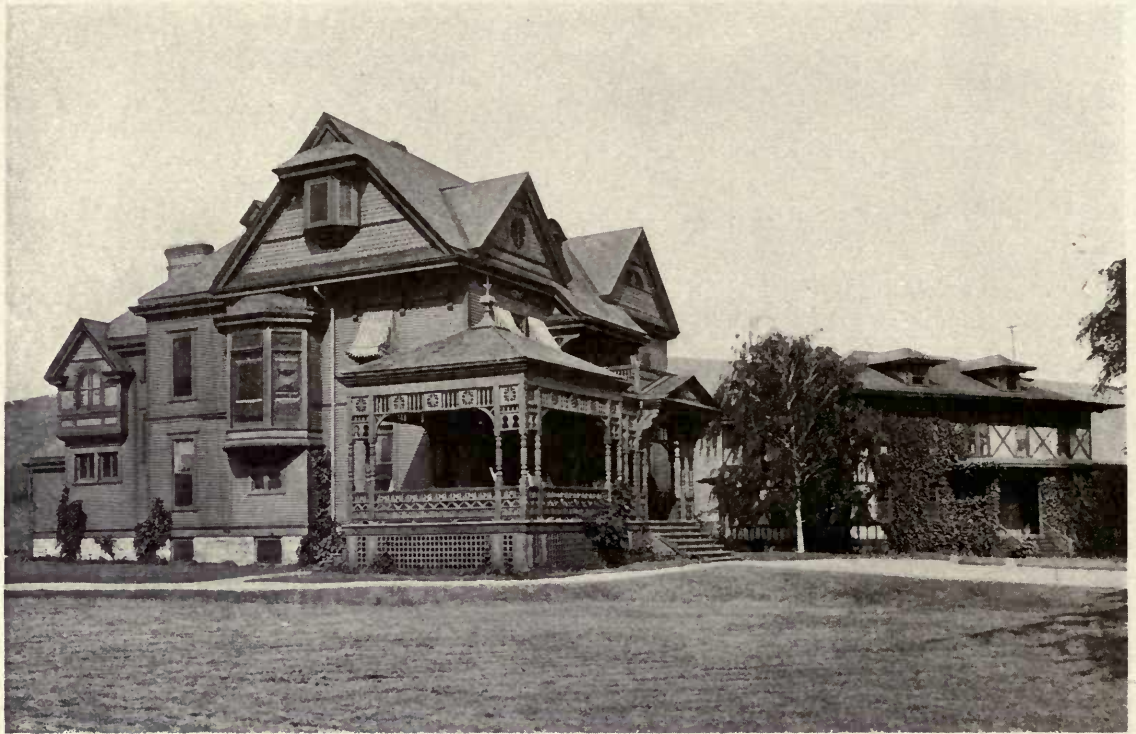
CLUB HOUSE AND DORMITORY
