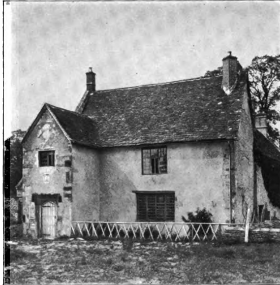
SULGRAVE MANOR HOUSE, NORTHAMPTONSHIRE.
