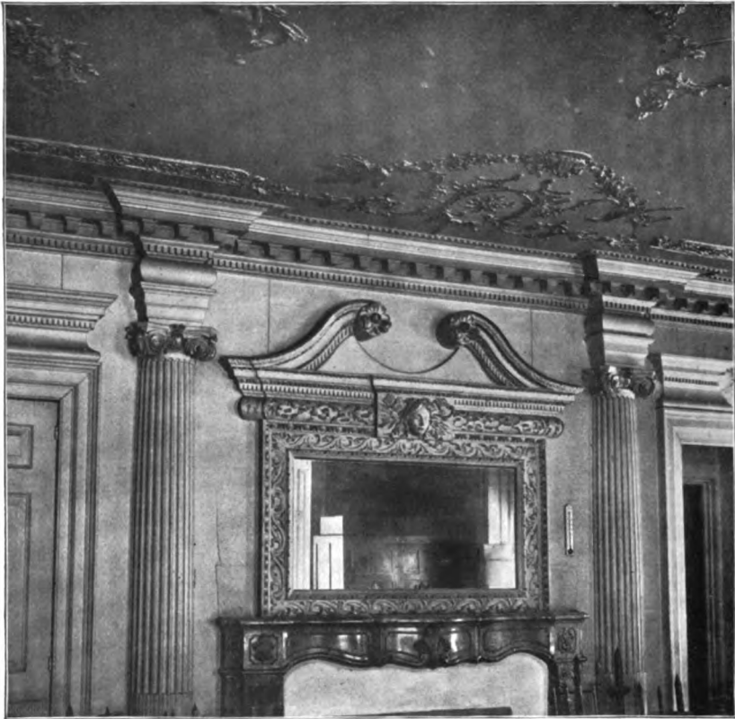
MANTEL AND CEILING IN DRAWING-ROOM, PHILIPSE MANOR-HOUSE.
