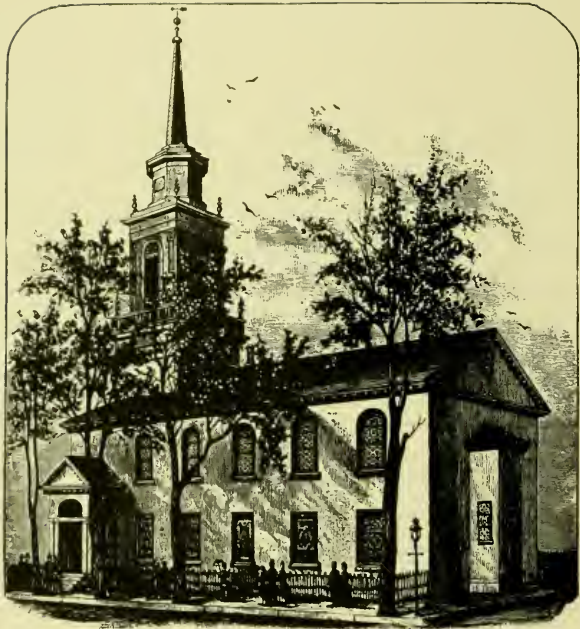
THE FIRST REFORMED CHURCH, EASTON, PA.
