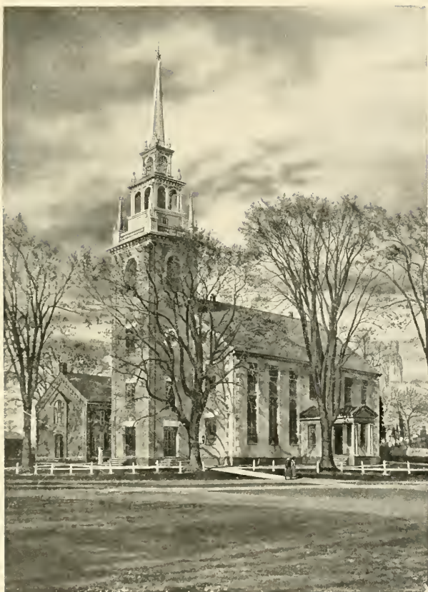
CONGREGATIONAL CHURCH, WETHERSFIELD, CONN. 1761
