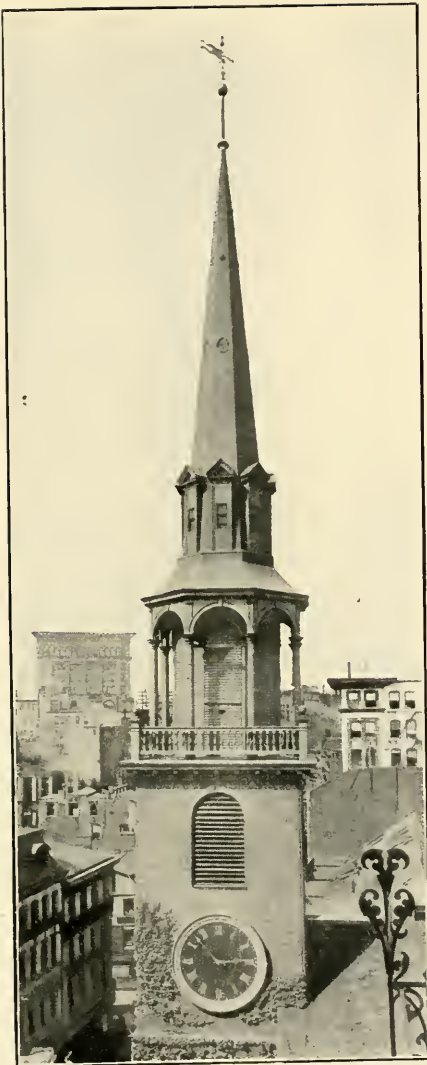
SPIRE OF THE OLD SOUTH CHURCH, BOSTON, WHICH HAD AN IMPORTANT INFLUENCE UPON LATER DESIGNS FOR CHURCH SPIRES IN NEW ENGLAND. CHURCH BUILT 1729
