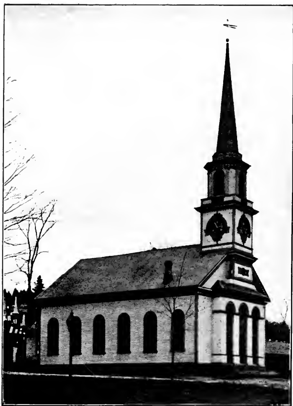
CONGREGATIONAL CHURCH, ENFIELD. 1787
