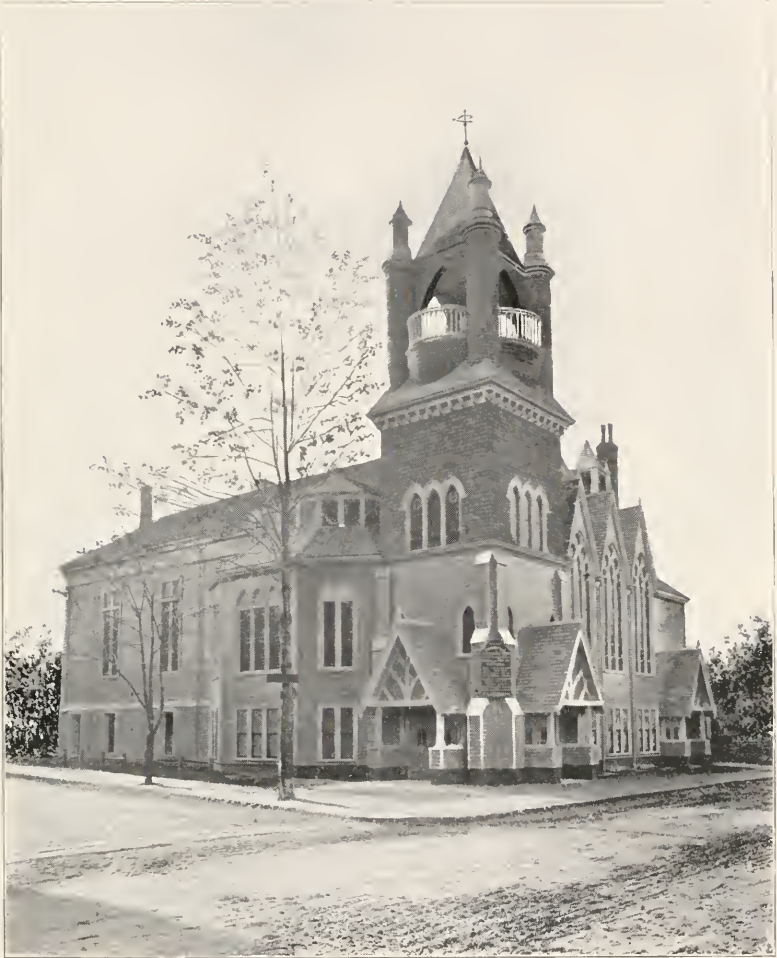
NEW DAY STREET CONGREGATIONAL CHURCH.
