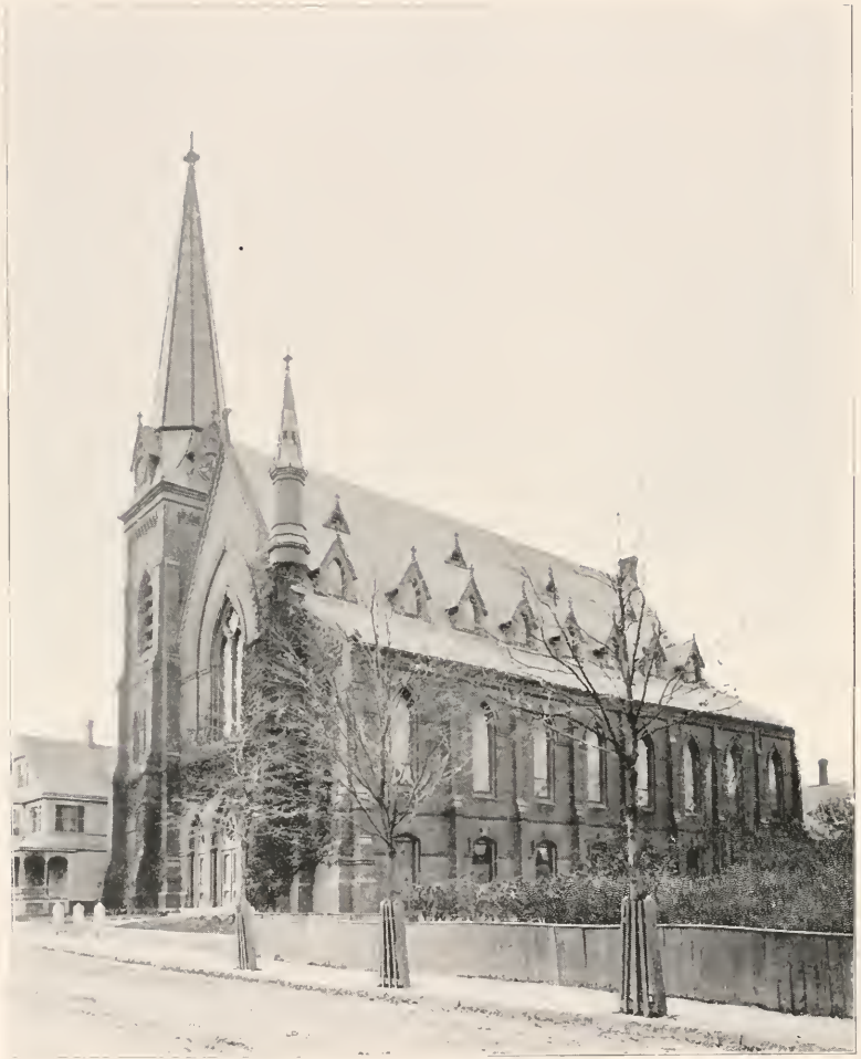
FIRST ORTHODOX CONGREGATIONAL CHURCH, Franklin, opposite Perkins Street.
