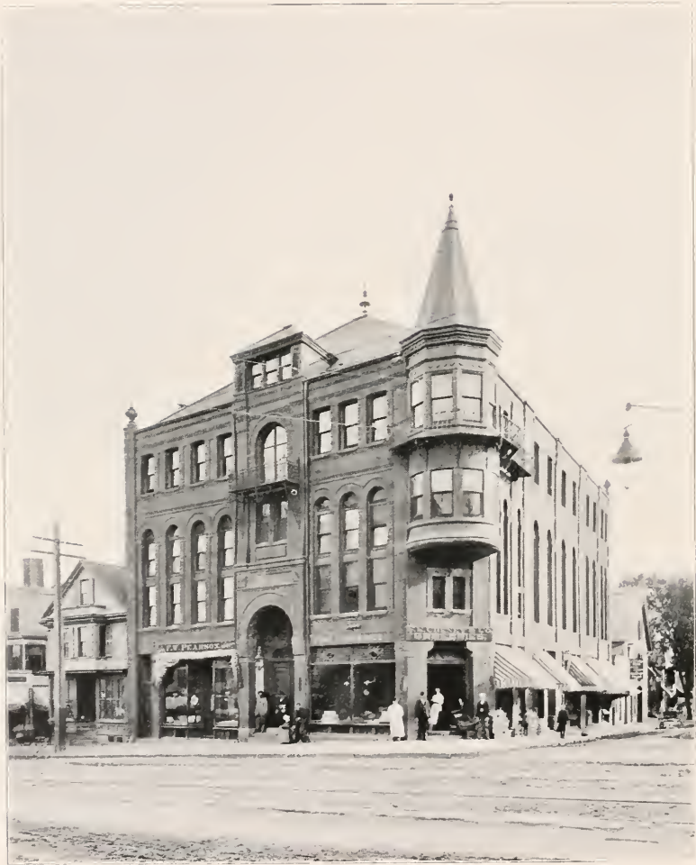
ODD FELLOWS' BUILDING, Broadway and Marshall Street.
