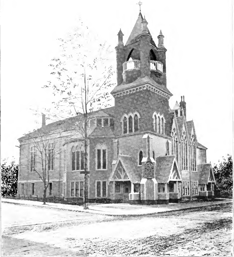
NEW DAY STREET CONGREGATIONAL CHURCH.
