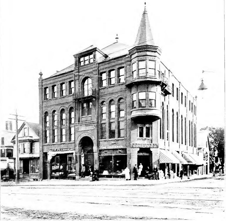
ODD FELLOWS' BUILDING, Broadway and Marshall Street.
