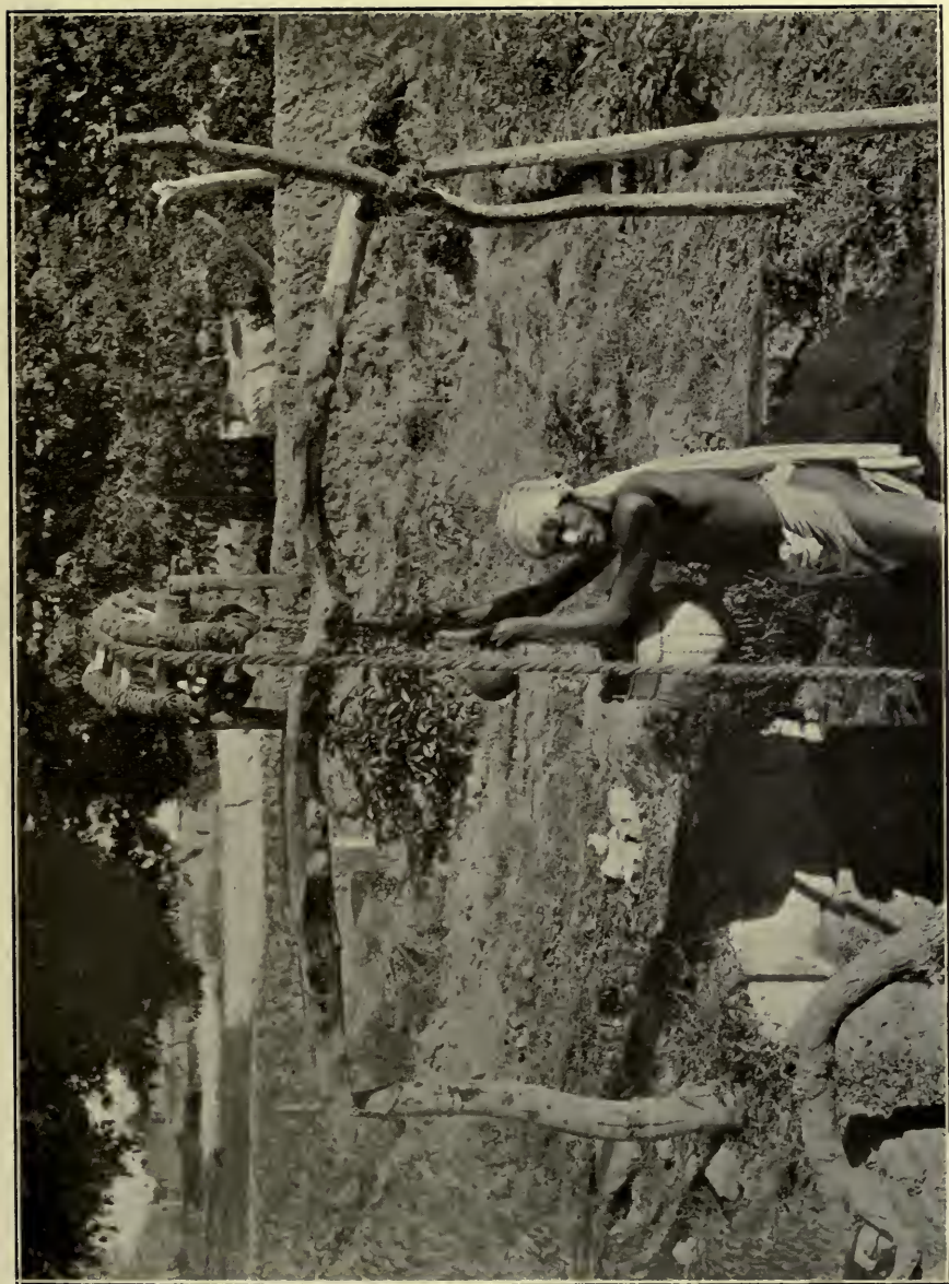
“RATANAM”, A FORM OF WATER-LIFT (TRUVALLUR).
