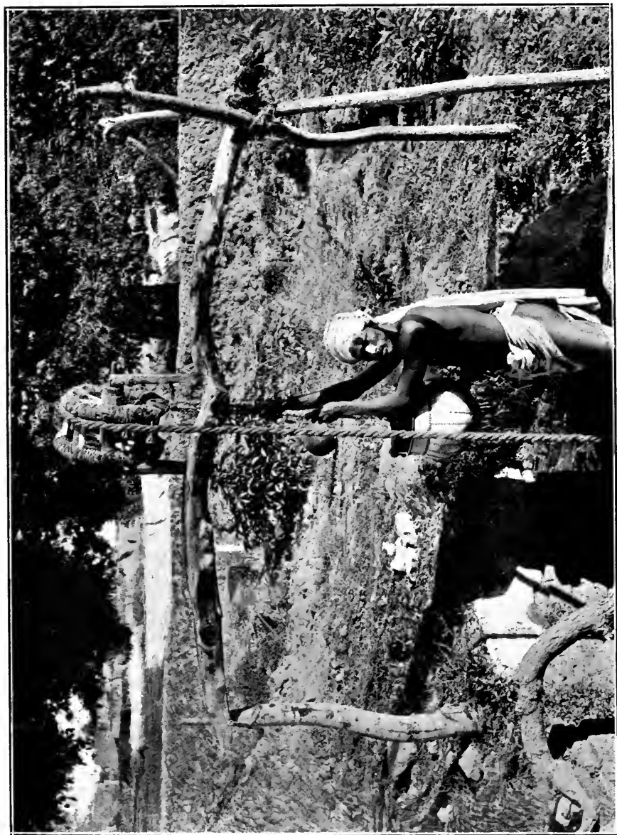
“RATANAM”, A FORM OF WATER-LIFT (TIRUVALLUR).
