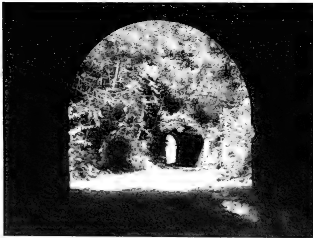
Fig. 15.—Culverts constructed of local limestone near Pearl, Pike County. These culverts supply the name—Twin Culvert Cave—for the nearby cave. An infrequently used county road and a small stream share the culverts.
