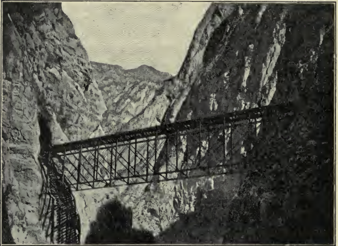
A BRIDGE IN THE MOUNTAINS.
