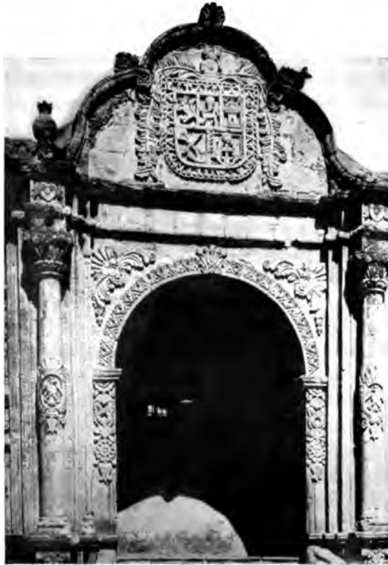
Ornamental Doorway of Oldest House in La Paz
