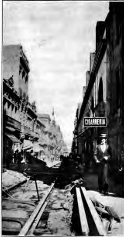
Street Scene, Montevideo. Laying of Car Track
