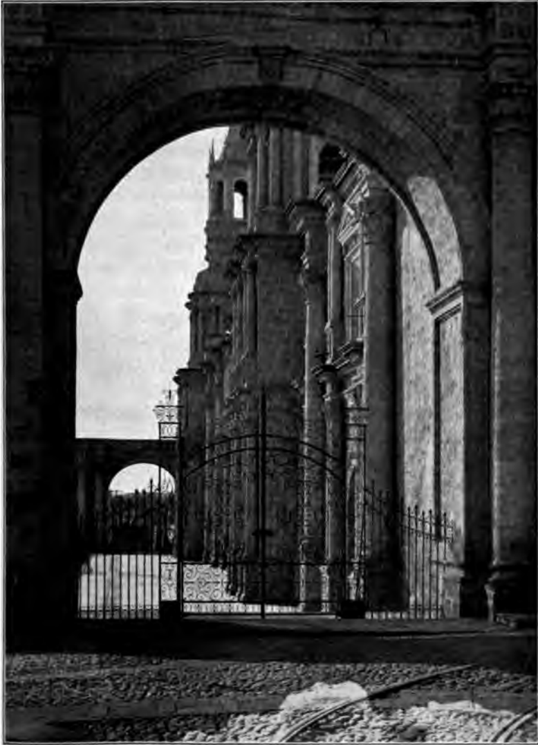
Side View of Façade, Arequipa Cathedral
