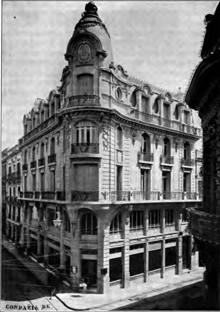
Life Insurance Company Building, Montevideo
