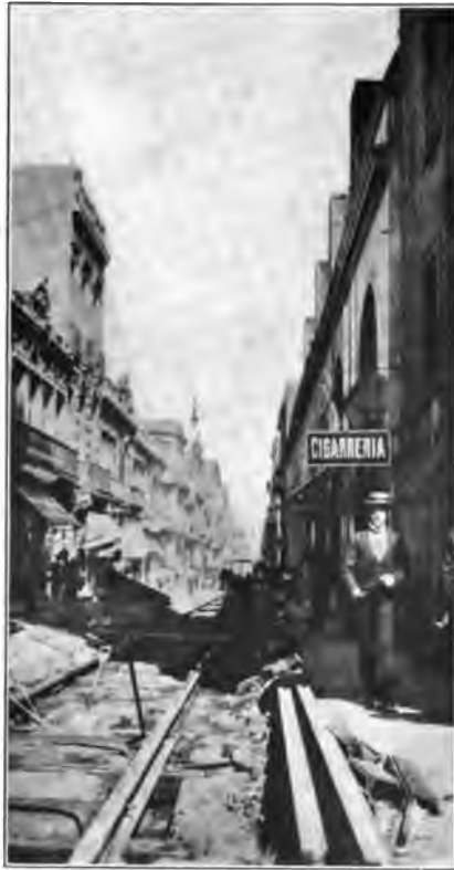
Street Scene, Montevideo. Laying of Car Track
