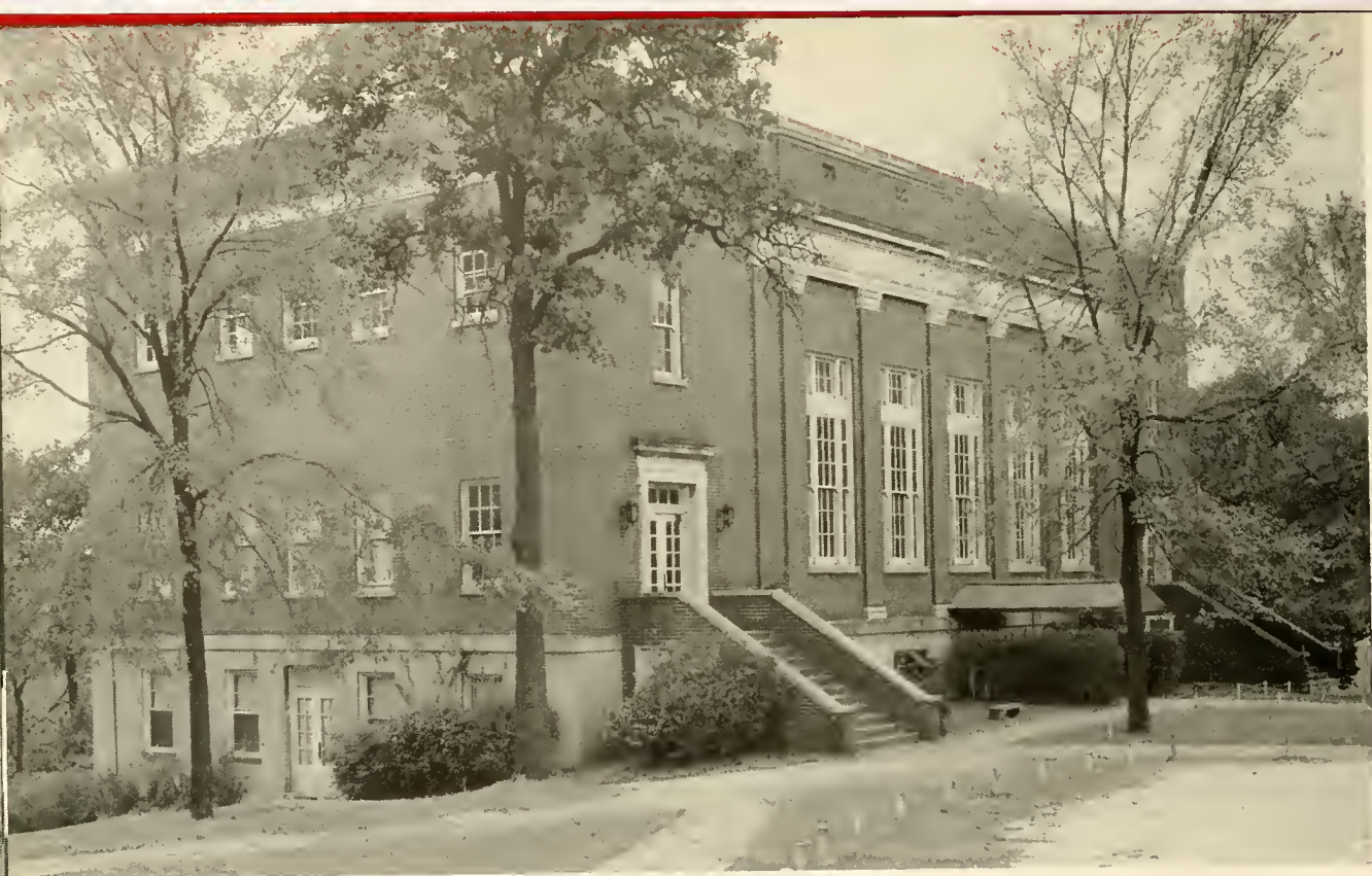
STUDENT ACTIVITIES BUILDING
