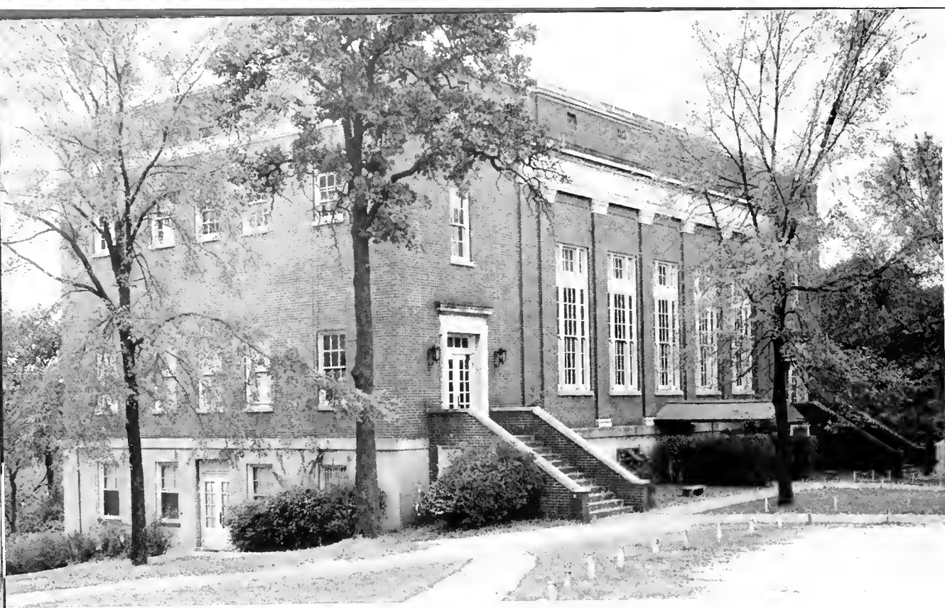
STUDENT ACTIVITIES BUILDING
