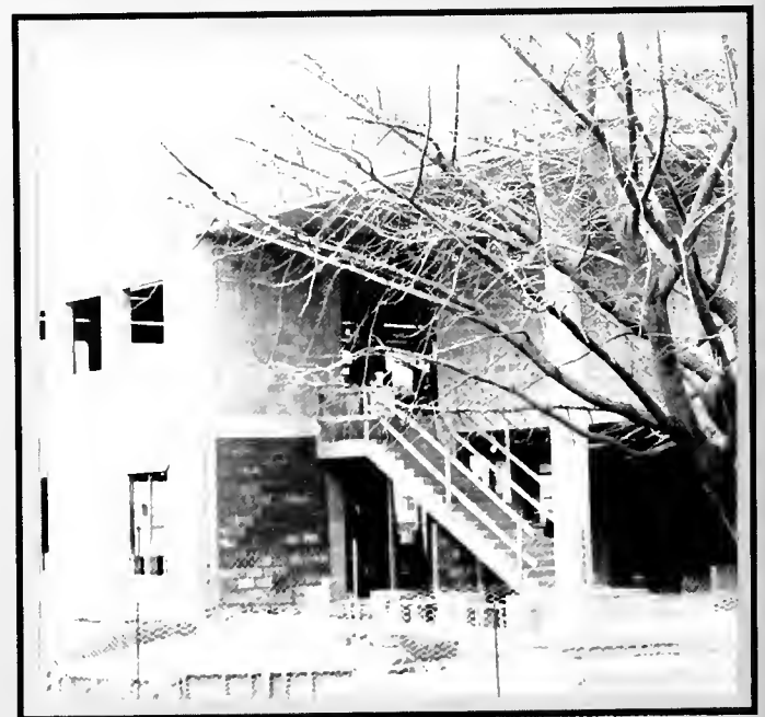
Even at this point in the construction, the annex's contemporary architecture is noticeable.
