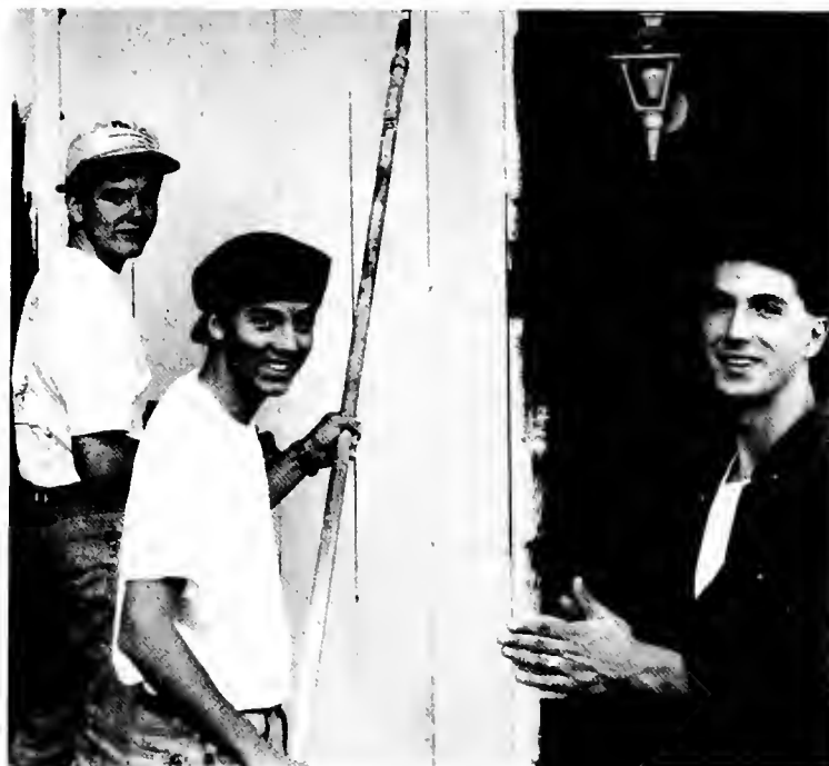
John Coley, Chris Rowell, and Jeff Jones also take part in repairing the Humane Society shelter.
