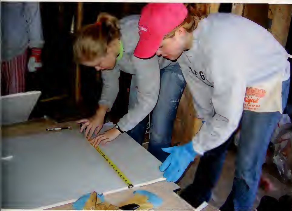
One of the most tedious tasks of the trip involves measuring the sheetrock to fit perfectly. This requires a lot of patience and many times must be performed several times to successfully complete. Miriam Smith and Susan Fant adhere to Stewart Jackson's advice: "Measure twice, cut once."
