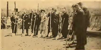
Members of the COMMITTEE OF 100 for progress and other dignitaries broke ground May 20 for the new physical education building at Southern Missionary College. The structure will cost approximately $200,000, exclusive of the swimming pool.
