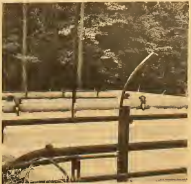
Pictured is part of SMC's new sewage plant completed at a cost of $165,000. These facilities, which will serve the major establishments on the campus, replace septic tanks and other obsolete methods.
