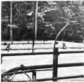
Pictured part of SMC's new sewage plant completed at a cost of $165,000. These facilities, which will serve the major establishments on the campus, replace septic tanks and other obsolete methods.
