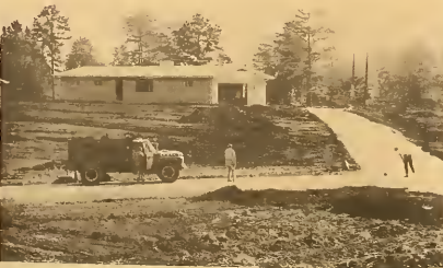
New home on Pierson Road nears completion.
