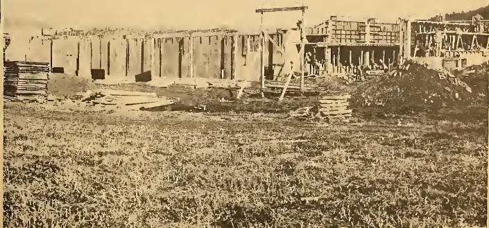
Foundation work nears completion on the $400,000 Collegedale Seventh-day Adventist Church.
