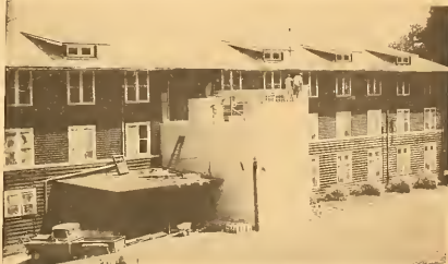
New bathrooms are added to Talge Hall.
