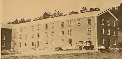
Outside work almost complete on WRH.
