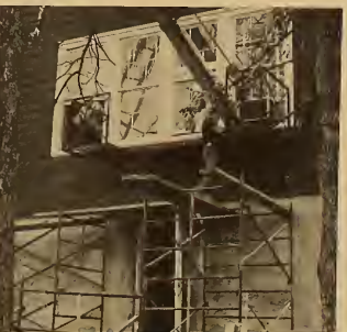
B and G workmen assemble the fire escape recently installed on the north end of Lynn Wood Hall.
