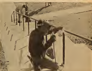
"A stitch in time saves nine." As the Buildings and Grounds Department employees stitched pipes together to make hand railings for various campus steps last week, SMC students were reminded of previous winters when students received the stitches instead of the pipe.
