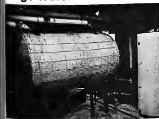
New 500-gallon holding tank installed in Talge Hall recently solves the hot water problem by supplementing the older heaters (right) and adding storage area.
