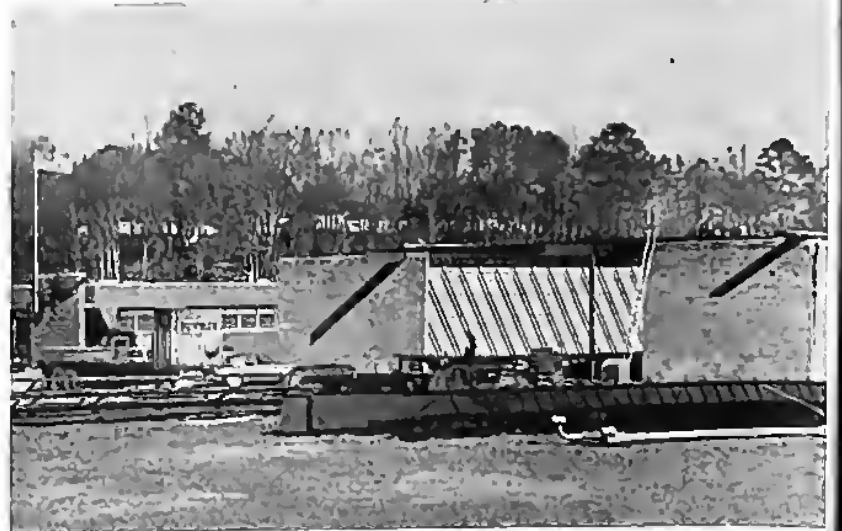
Construction on the new College Plaza supermarket begins again after a brief lull.
