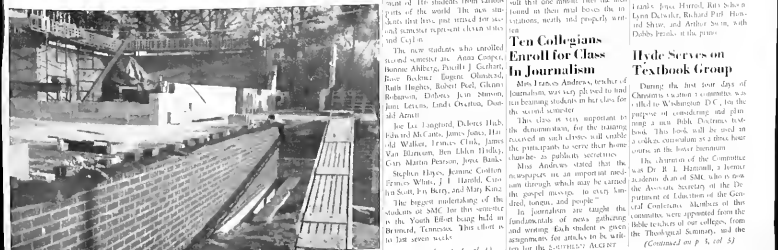
Work is progressing on the new Home Economics Building.
