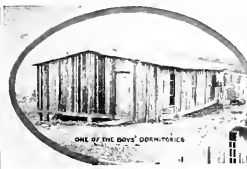
The First Boys' Dormitory.
