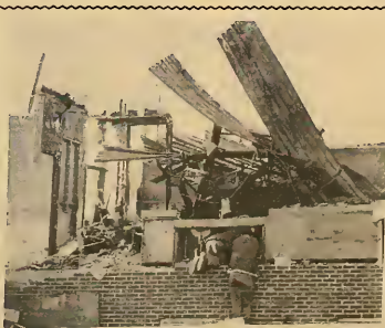
A fire gutted the A.W. Spaulding Elementary School's auditorium on February 6.
