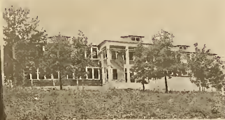
A windowless Lynn Wood Hall as it appeared during construction, circa 1924
