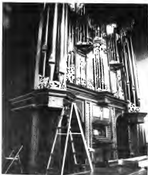
Repairs on the organ should be completed by mid June.
