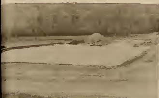
Construction has finally begun on the long-promised sandpit volleyball courts.
