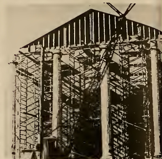
Wright Hall under construction in 1967.
