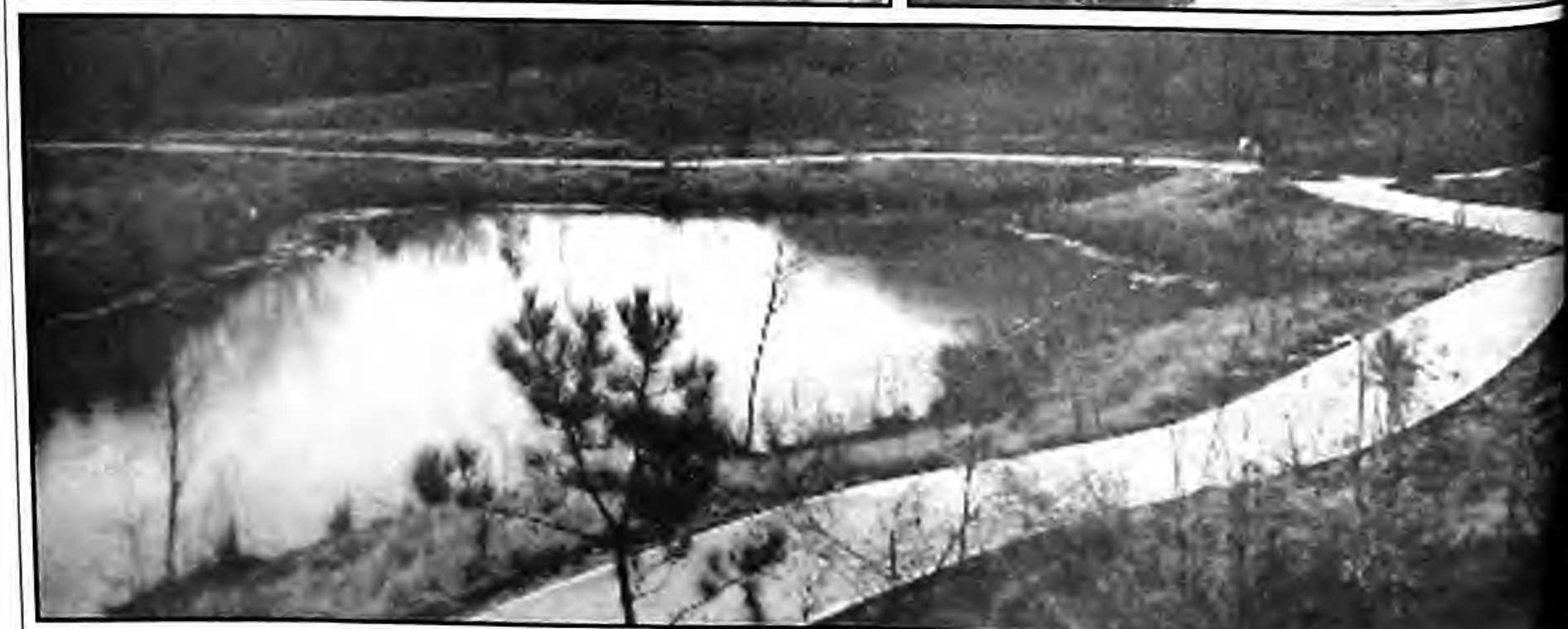
The Wolftever Greenway (top left) starts behind Collegedale City Hall at Imagination Station, crosses under Ooltewah-Ringgold Road (top right) and circles a wetlands pond (above). The trail is nearly a mile long. Construction volunteers include students and faculty from A. W. Spalding Elementary and Collegedale Academy. While the Greenway is open, the ribbon-cutting ceremony will not be celebrated until next Sunday, March 28, at 2 p.m.
