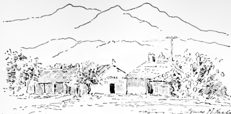
Adobe buildings near Pala Mission.
