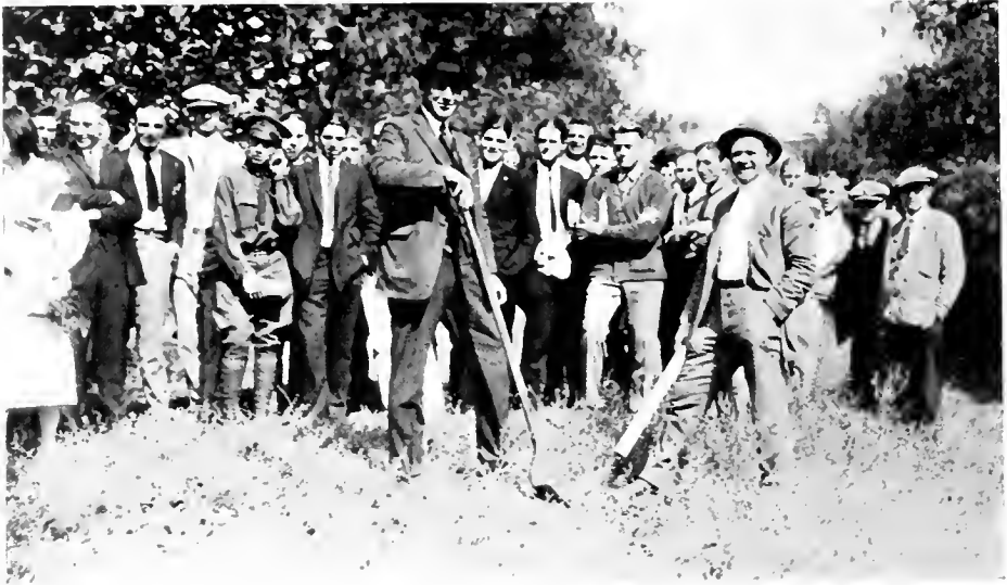
BREAKING GROUND FOR THE SWIMMING POOL
