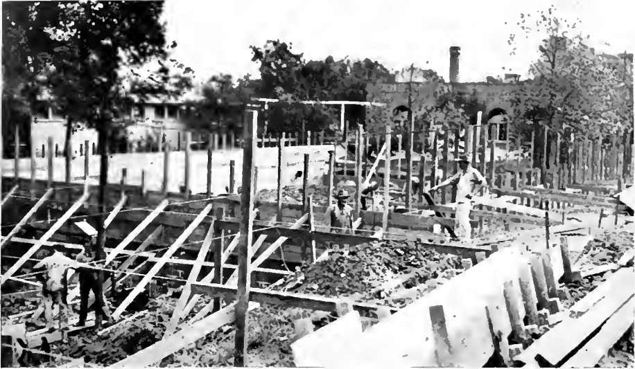
SWIMMING POOL DURING CONSTRUCTION
