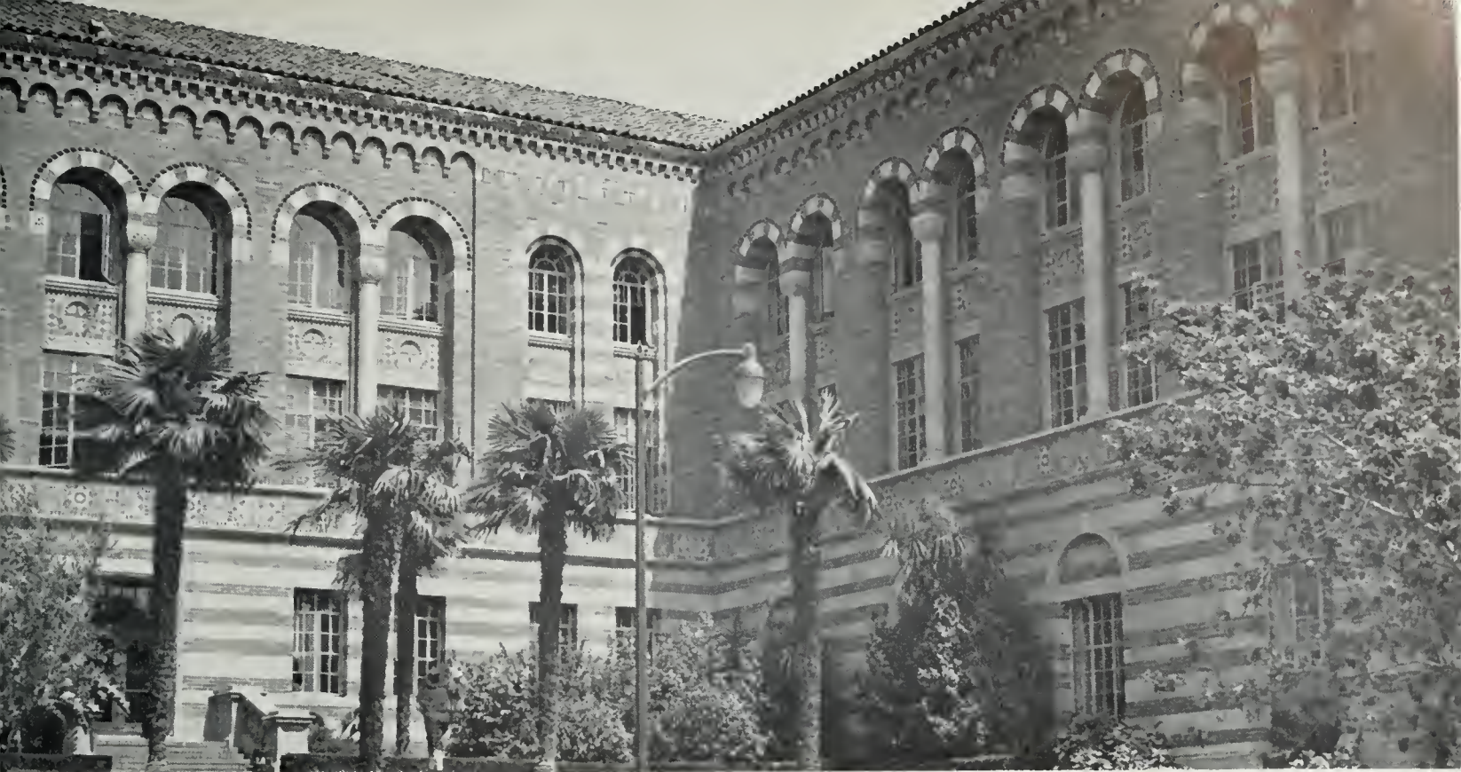
ONE OF THE FIRST BUILDINGS CONSTRUCTED AT UCLA, MOORE HALL PROVIDES CLASSROOMS FOR EDUCATIONAL COURSES AND BOASTS BOTH A NEW LOUNGE AND LIBRARY.
