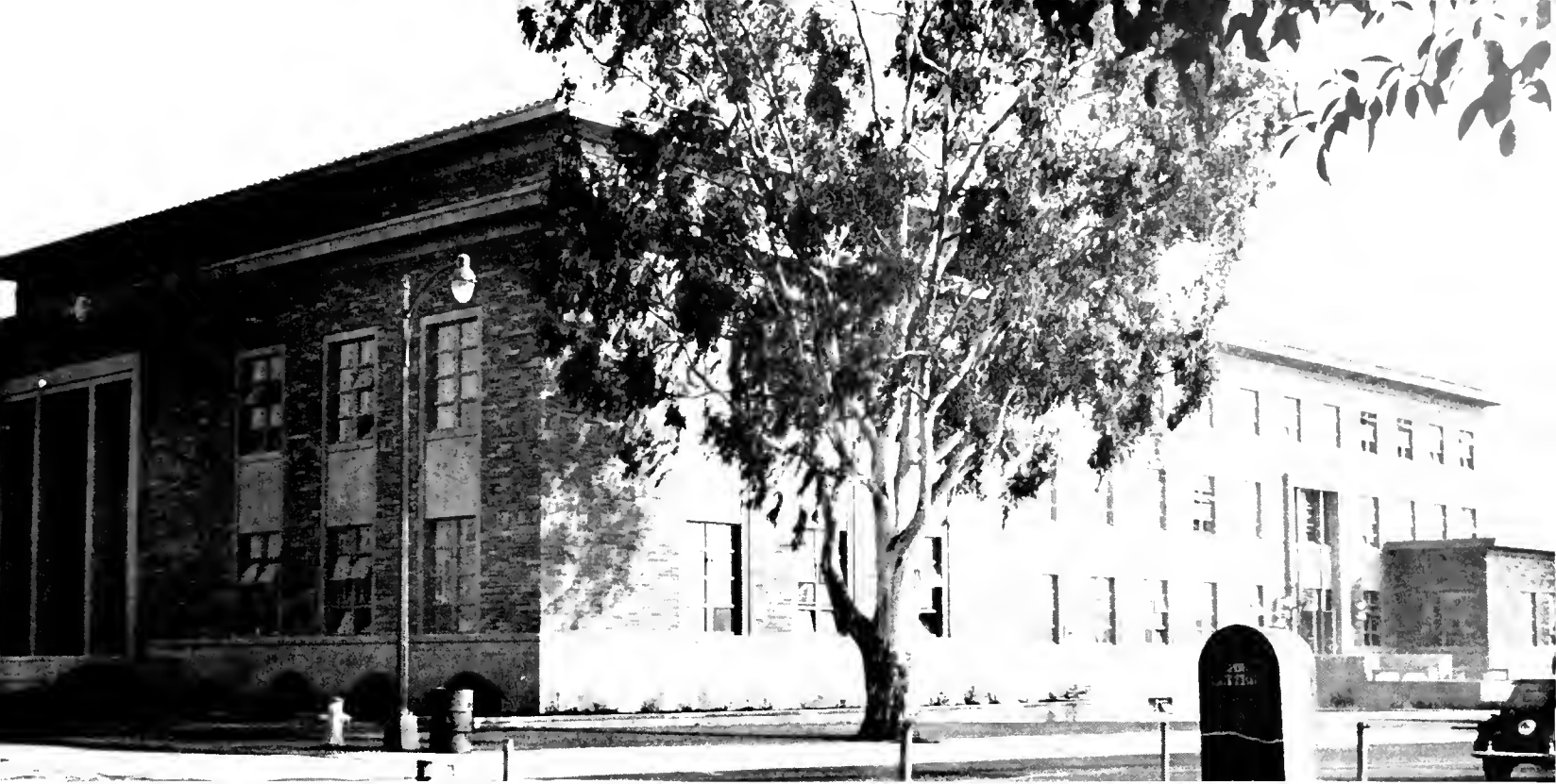
NUCLEUS OF ACADEMIC MATTERS, THE ADMINISTRATION BUILDING CONTAINS OFFICES OF THE PRESIDENT, CHANCELLOR, REGISTRAR AND DIRECTOR OF ADMISSIONS
