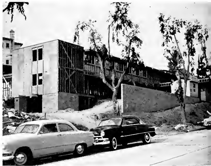
The long awaited Sigma Chi house, which was completed in the fall, features the latest in modern architecture and design.
