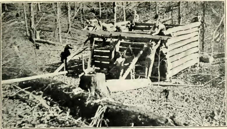
"Raising a house"—Rolling a Log up Over the Skids into Position
