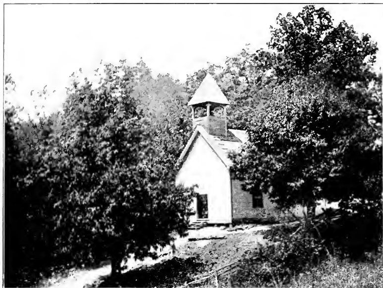
Mountain Church and School House
