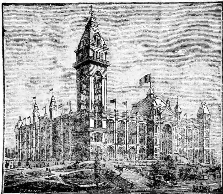
New Factory Building Just Purchased By INTERNATIONAL STOCK FOOD CO., Minneapolis, Minn.
