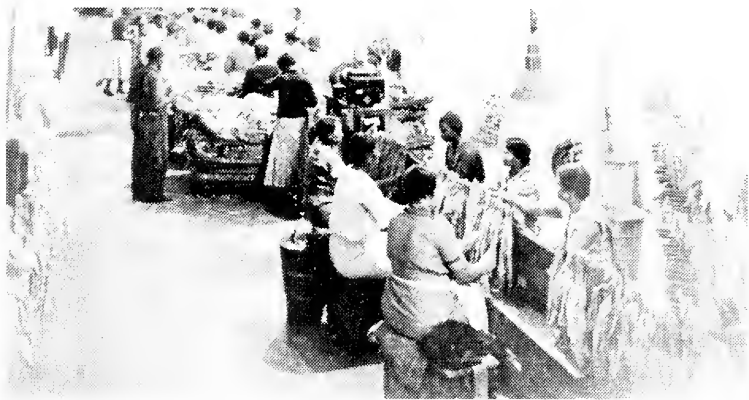
African American employees hanging tobacco in a stemming and redrying plant, Kinston, North Carolina, 1935 [courtesy of North Carolina Collection]
